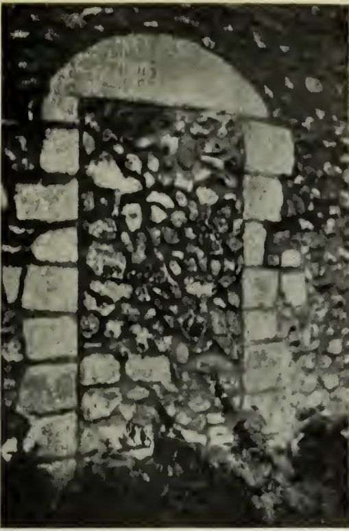
STURMER CHURCH. North doorway of nave ; 11th-century.
